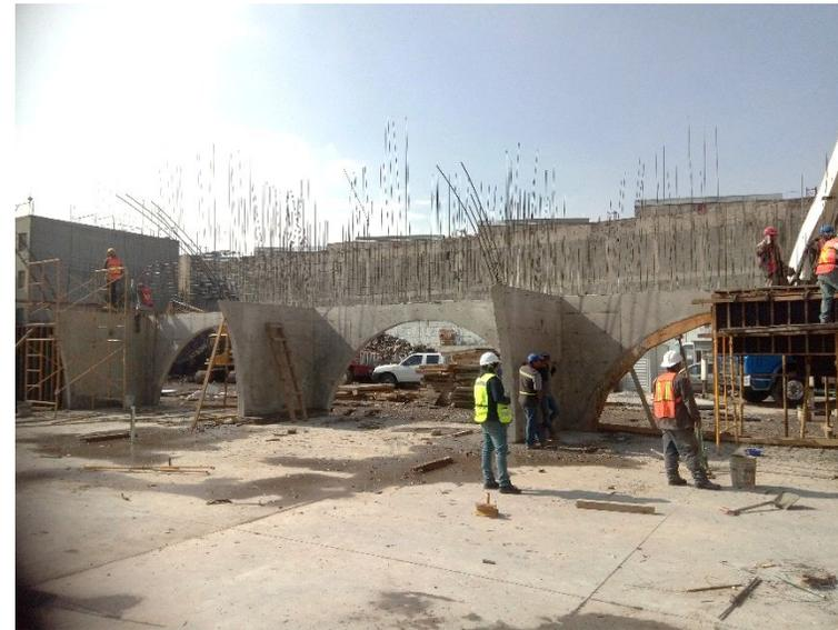
**COLADO CON CONCRETO PREMEZCLADO  $F'_{C}=250\text{KG}/\text{CM}^2$
