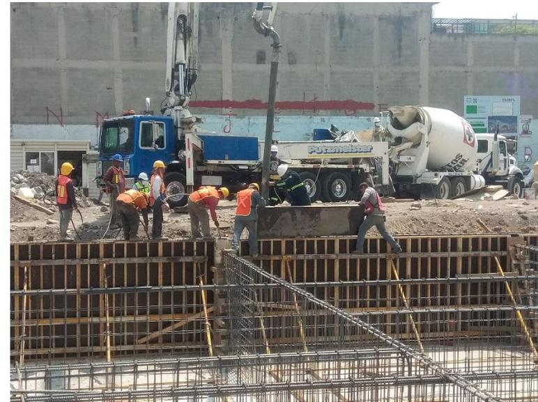
**COLADO CON CONCRETO PREMEZCLADO F'C=250KG/CM2 PARA MUROS MC-1
