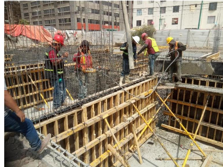
**COLADO CON CONCRETO PREMEZCLADO F'C=250KG/CM2 PARA LOSA Y MUROS MC-1/MC-2
