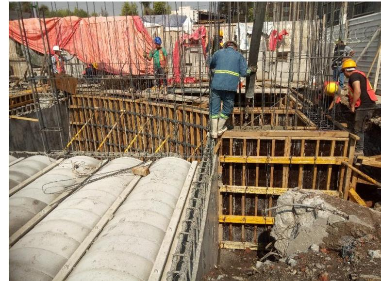
**COLADO CON CONCRETO PREMEZCLADO  $F'c=250\text{kg/cm}^2$  PARA MUROS MC-1/MC-2 DE LA CIMENTACION DEL EDIFICIO PRINCIPAL (EJES 1-2/B-C)**
