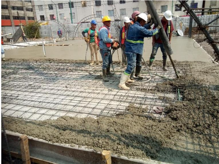
**COLADO CON CONCRETO PREMEZCLADO F´C=250KG/CM2 EN
